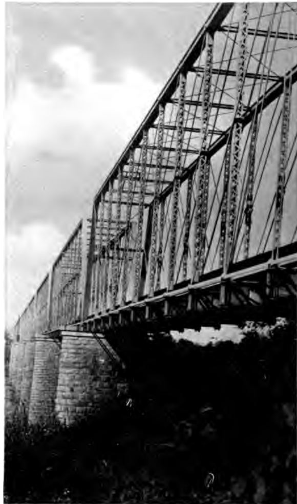
TENNESSEE RIVER BRIDGE. Eight spans. Total length, 1204 feet; height above low water, 63 feet.
